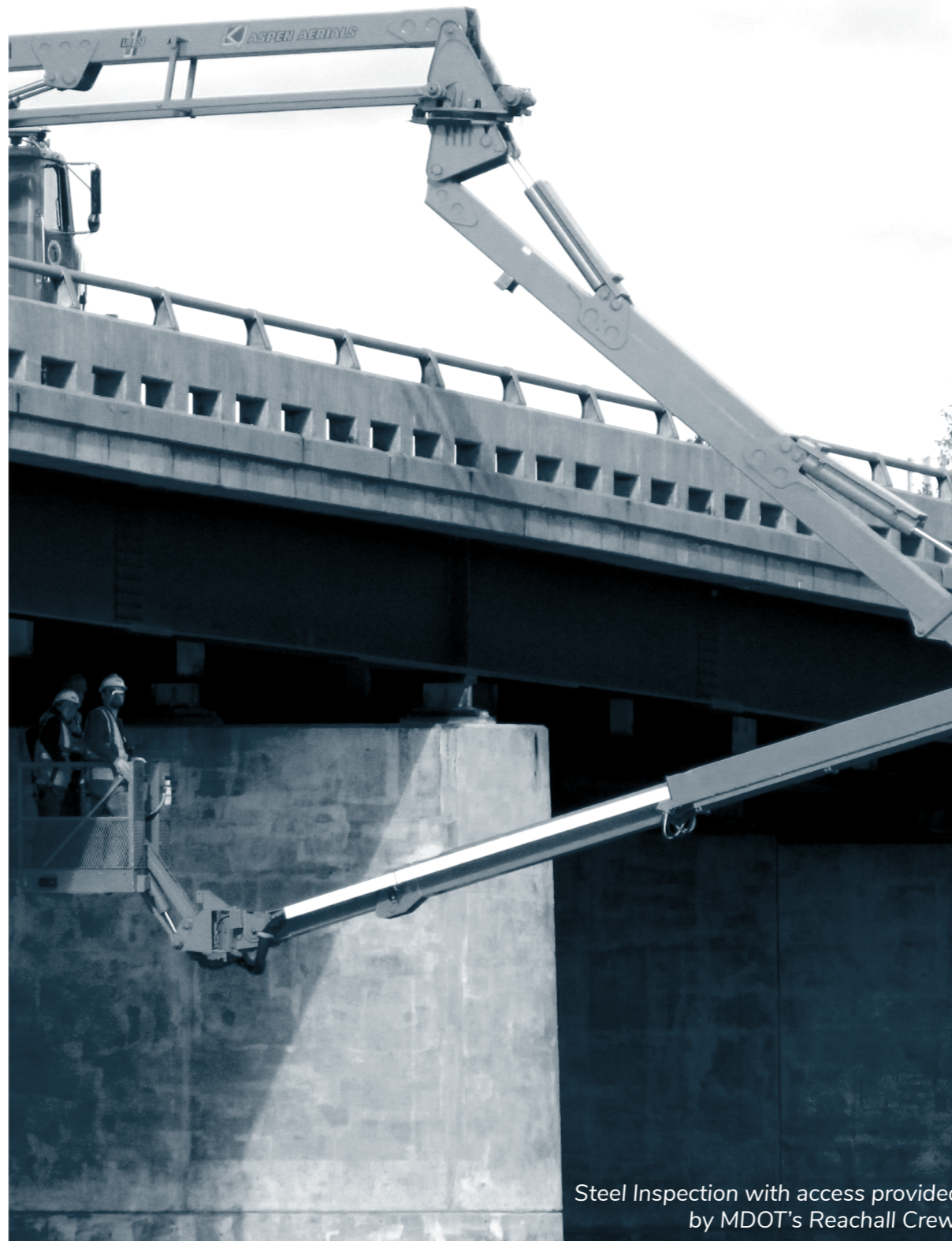
Spicer Group crew members sounding concrete checking for delaminations on bridges in Battle Creek along I-94.
