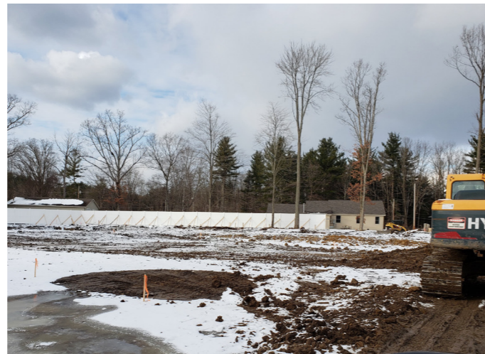
New site cleared and ready for construction.
