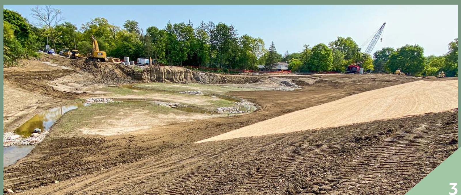
Photo 3 - Floodplain excavation continues, preparing for outlet control structure installation
