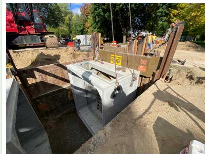
Downstream end of outlet control structure
