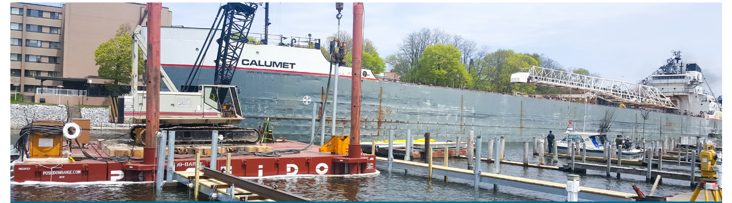
Freighter coming through the Manistee River during construction.
