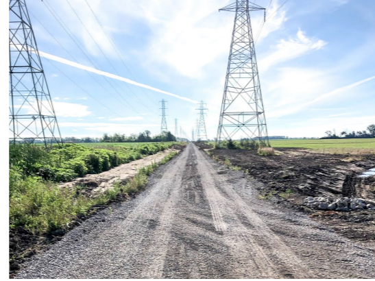
Gravel along the pathway before pavement during construction.
