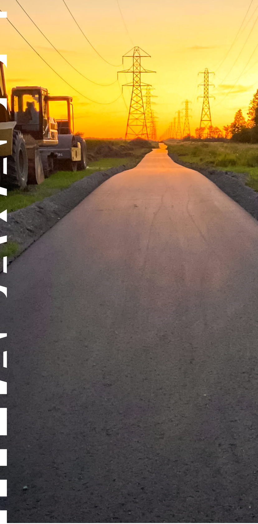
The newly finished Tittabawassee Township pathway near Garfield Road at sunset. Photo by Andy Brady of Dig Deep Race Events.
