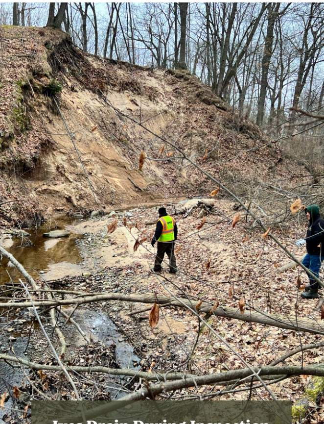
Ives Drain During Inspection
